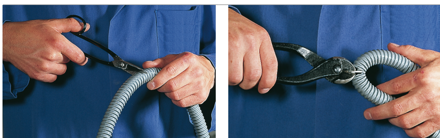
Kunststoff-Ummantelung durchschneiden Cut through the plastic sheathing
